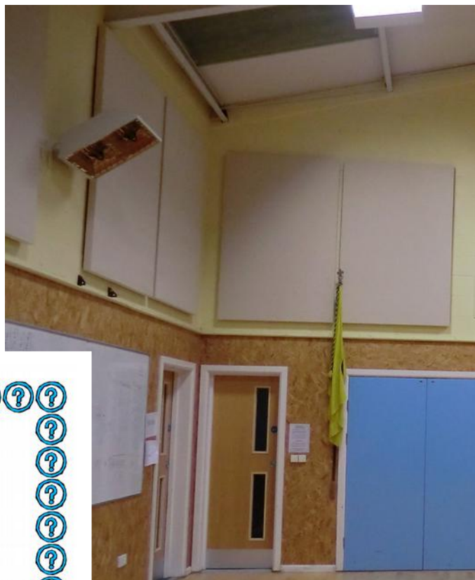
Above: New acoustic panels in the H.Q.
